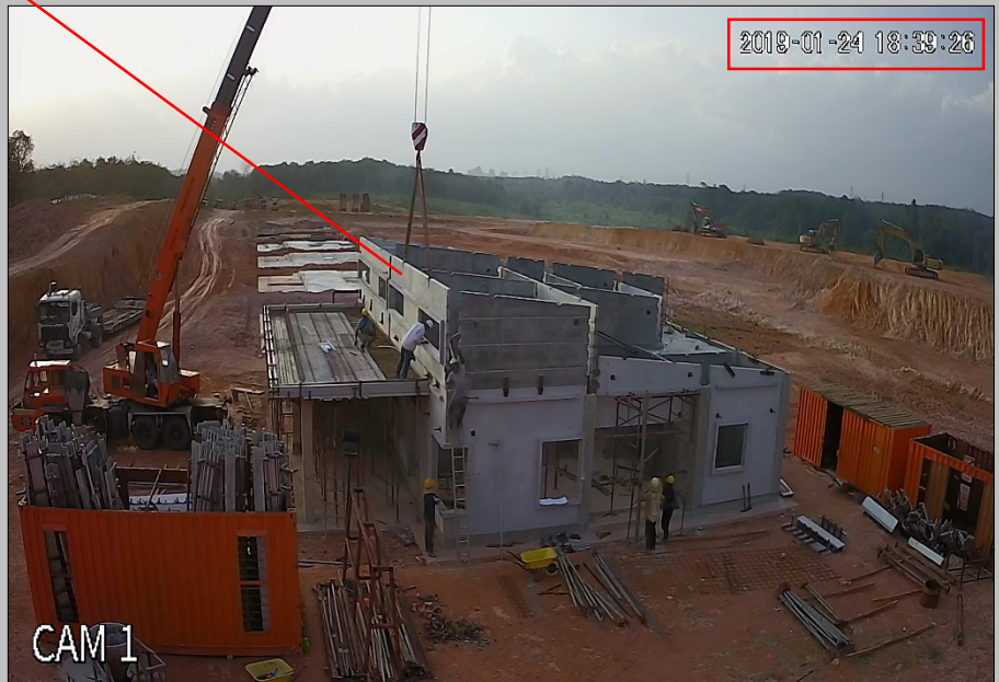
- Precast wall panel installation
