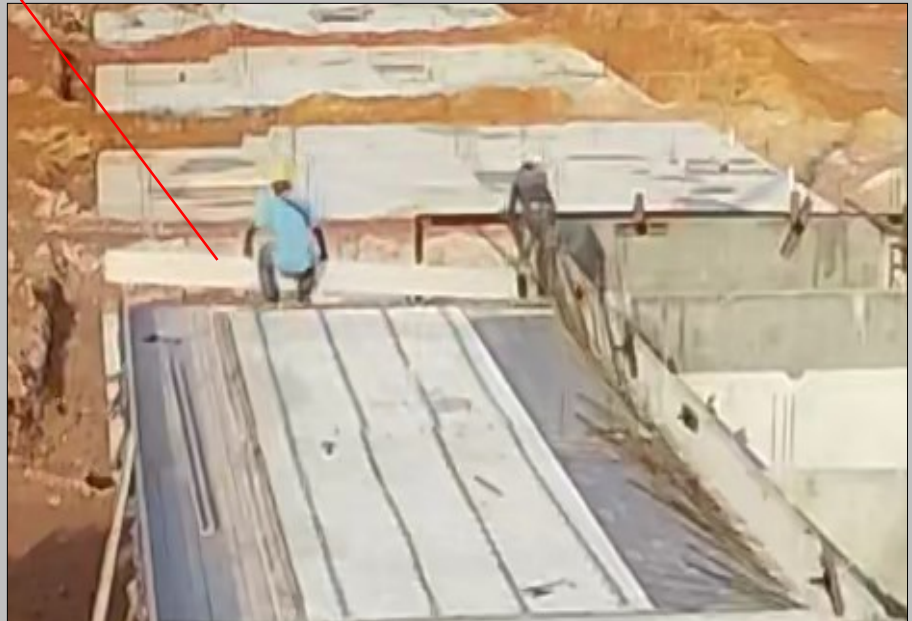
- In-situ coping modular mould installation
